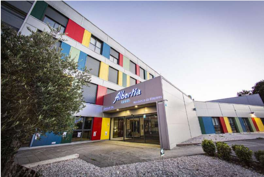
Fig. 14. Albertia Group's Residence in Lugo
