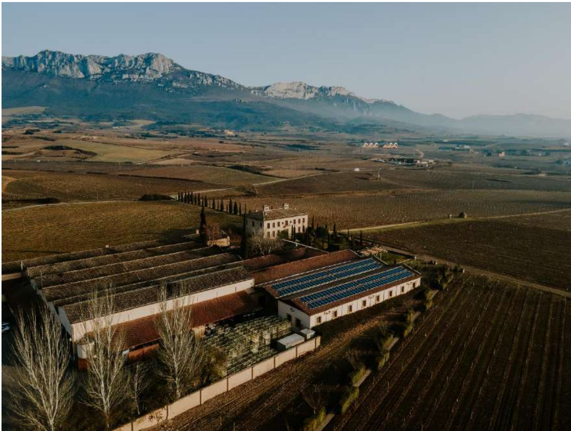
Fig. 16. Solar Panels in Torre de Oña
